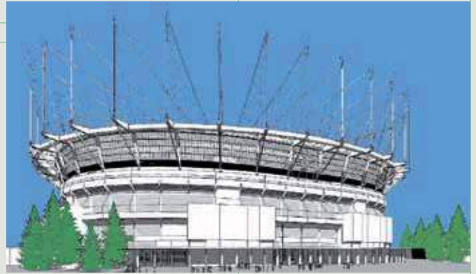
BC Place stadium, Vancouver (Canada) – 2010/2011 – Freyssinet/Advitam Renovation of the suspended roof and installation of Advitam’s sensors to monitor, among other tasks, real-time load and vibration influencing a structure’s stays, ensuring that it stays in good condition.
