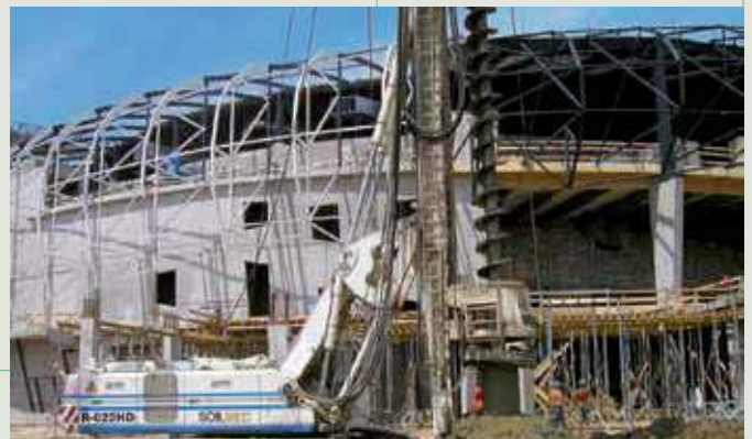
Budapest Arena (Hungary) – 2001 – Soletanche Bachy Use of a hollow stem auger to create 17,000 ml of piles.
