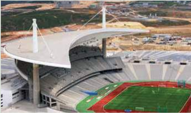
Ataturk Olympic stadium (Turkey) – 2001 – Freyssinet Four Freyssinet stays support the roof in the shape of Turkey’s national symbol, the crescent.
