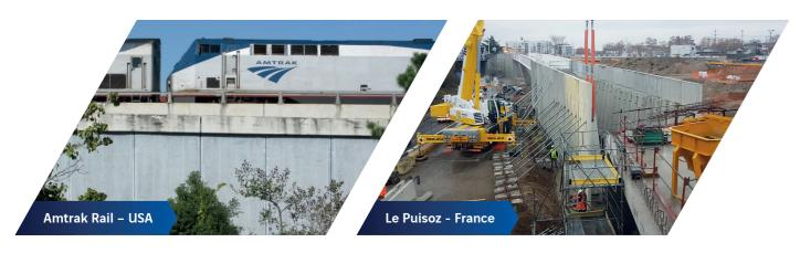
TechWall™ relies on counterforts, which play a crucial role in ensuring the overall stability and strength of the retaining wall. By acting as cantilever beams, the counterforts can effectively resist the lateral earth pressure, thereby reducing the moments in the facing panel. As a result, the thickness of the concrete panel can be minimized, without compromising the strength and durability of the structure.
